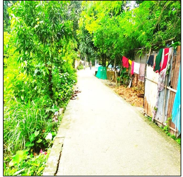
Drain- 19, Kumarkhali Pourashava
